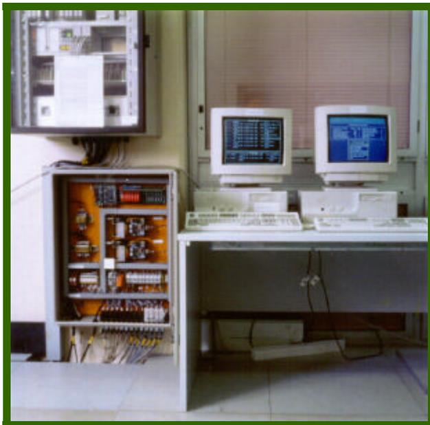
This photo shows the control cubicle (designed by Holman Engineering) with the door open on the bottom left, the Alarm Interface computer in the middle, and the file server computer on the right hand side.
