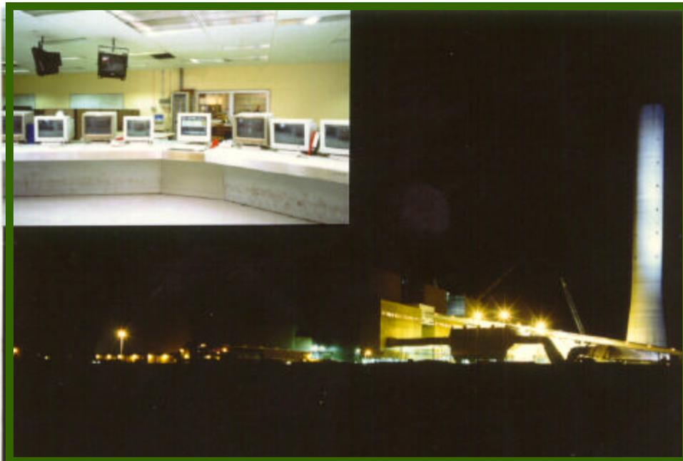
Above is a photo of the Stanwell power station at night, with the insert being a photo taken inside one of the two control rooms at the power station. The computer in the centre of the control desk in one of the man/machine interfaces for the PPAI system.
